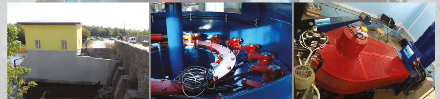
Delivery and installation of a turbine at Gubyn hydroelectric power plant (Ukraine)
