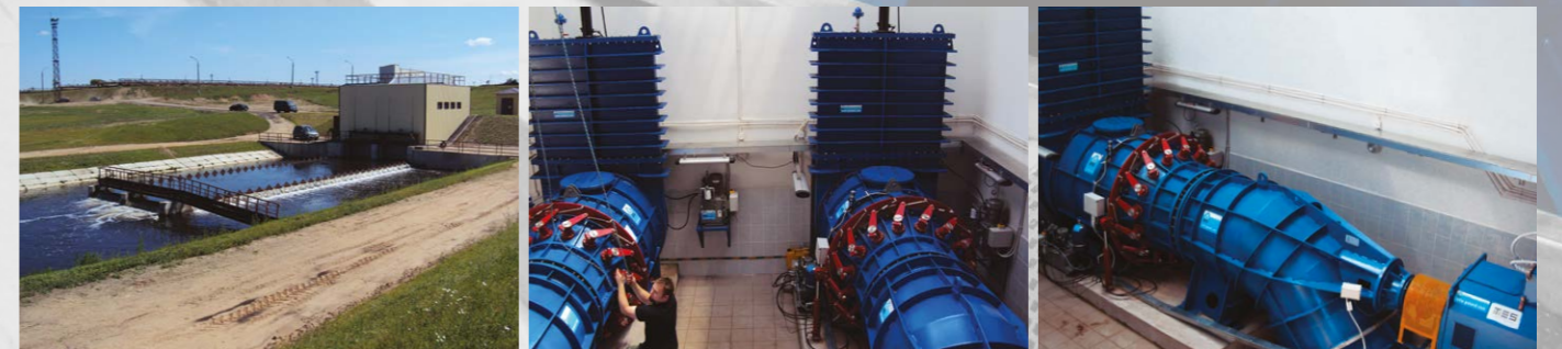
Delivery and installation of a turbines power 2 x 412 kW at Szabany hydroelectric power plant (Belarus).
