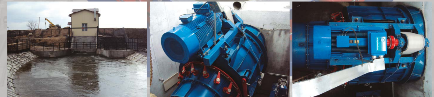
Delivery and installation of a turbine at Staraya Chortoriya hydroelectric power plant (Ukraine).
